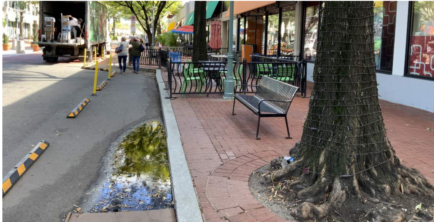
Unsafe and insufficient space for pedestrian circulation
